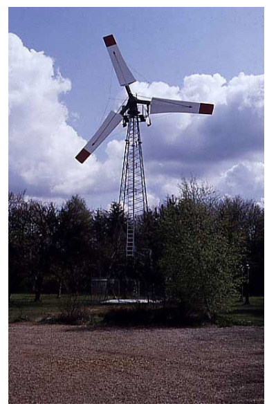
Green Mountain Power is currently constructing a wind turbine field in
